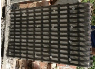
Figure 1. External strengthening of the wall with SGU300 grade geo-grid
